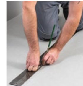
1. Clean and mark out the installation area
