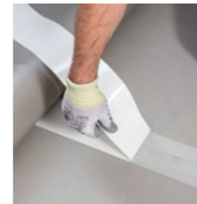
3. Remove the protective film then roll out the flooring
