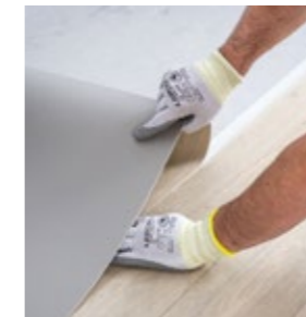
3. Remove the protective film then roll out the flooring
