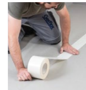
2. Install the hop holding tape & position the strips
